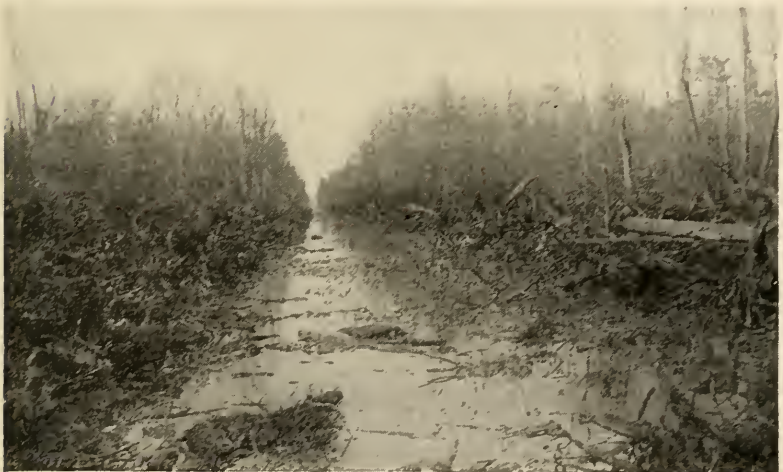
FIG. 100.—A neglected ditch often seen in heavily wooded areas. (H. C. Wheeler.)
